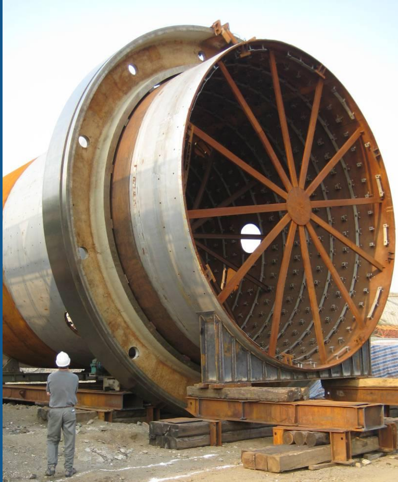
Support Tyre Placed on Outer Shell (Shell Fabricated in China, Tyre Cast in Czech Republic)
