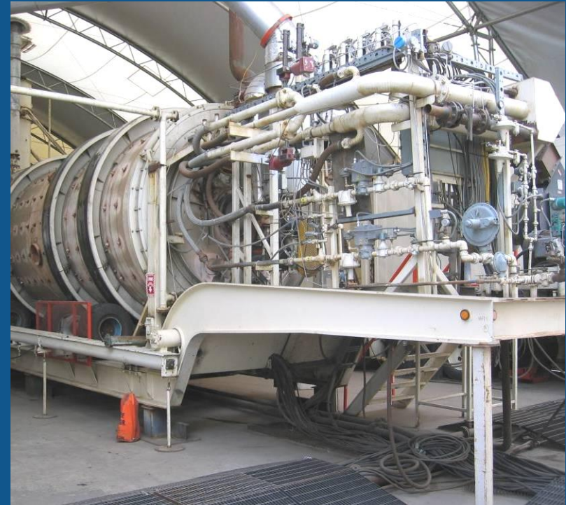
ATP60 Pilot Plant
