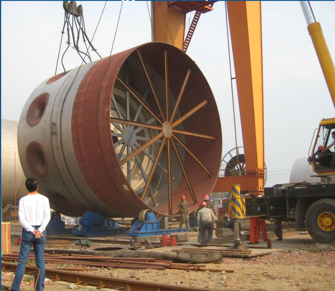
ATP Processor Erection in China September 2008
