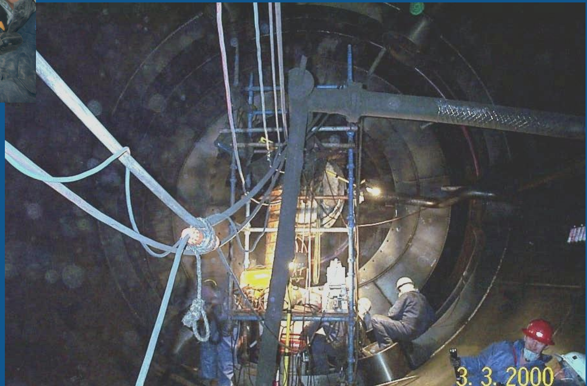
Six People Working in the Stuart Demonstration Plant Retort Zone
