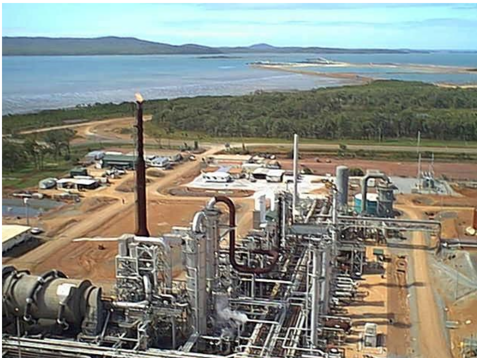
The Stage 1 ATP Demonstration Plant at the Stuart Project in Australia (Processor at lower left)
