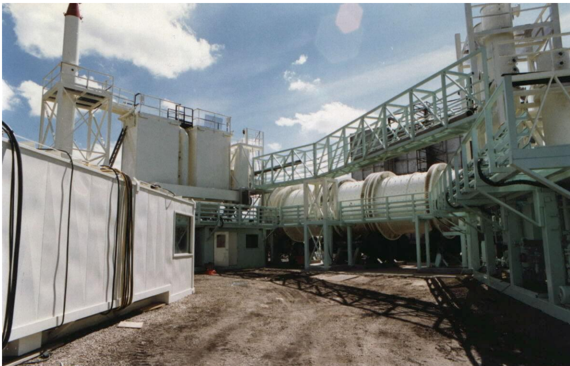
The 10 t/h ATP Plant at a U.S. EPA Superfund Site in New York
