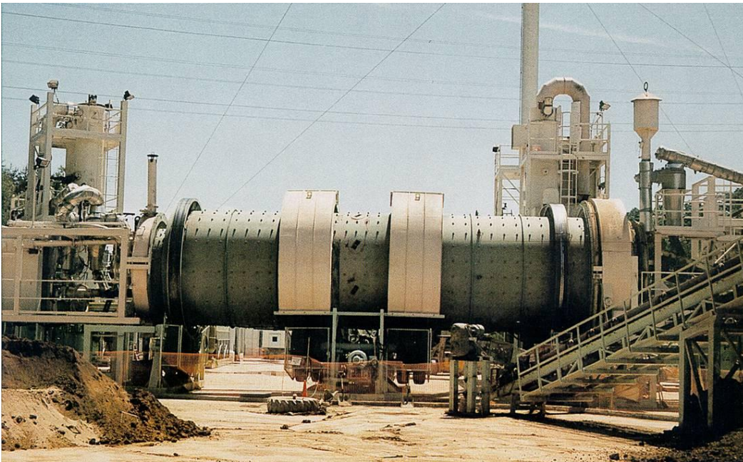
The 10 t/h Feed Capacity ATP Processor at a Superfund Site in the USA
